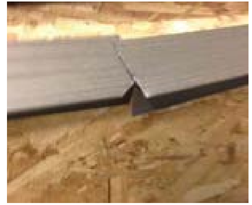
3. Sometimes the bottom hem will also need to be cut to make sure there is a tight fit. Screws should be in the middle of the width halfway up the roof.
