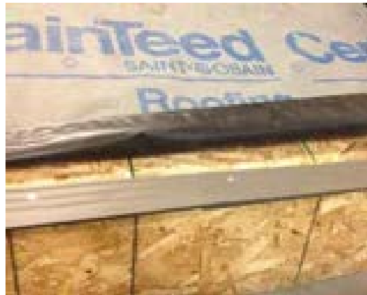
4. After the drip edge is completely installed on eaves, install MetaLayment/WinterGuard® HT over the drip edge in accordance to local building codes, followed by DiamondDeck®.
