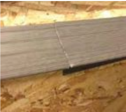
4. After the drip edge is completely installed on eaves, install MetaLayment/WinterGuard® HT over the drip edge in accordance to local building codes, followed by DiamondDeck®.
